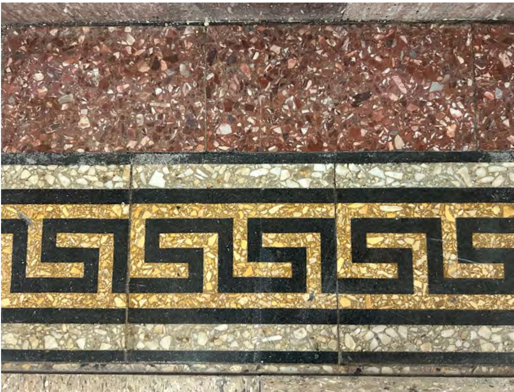
17. Capitol (1900), second floor, uncovered section of terrazzo floor, photographer facing east.
