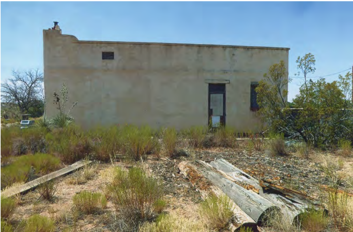
North side, photographer facing south.
