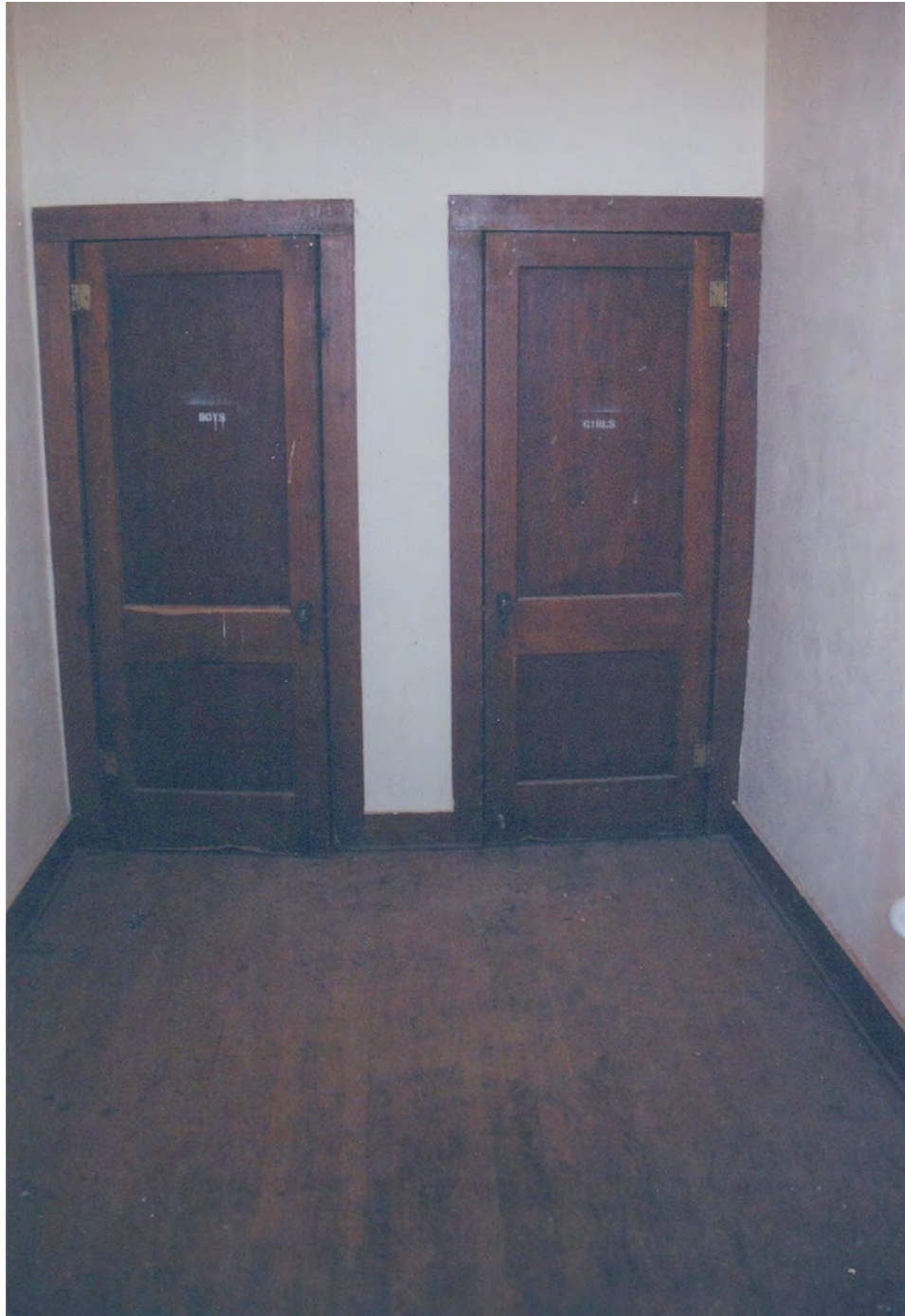
Main corridor, boys' and girls' restrooms, photographer facing west.
