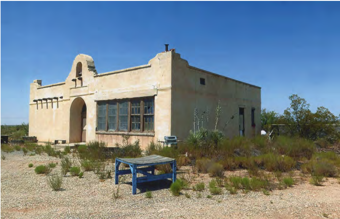
Main façade and north side, photographer facing southwest.
