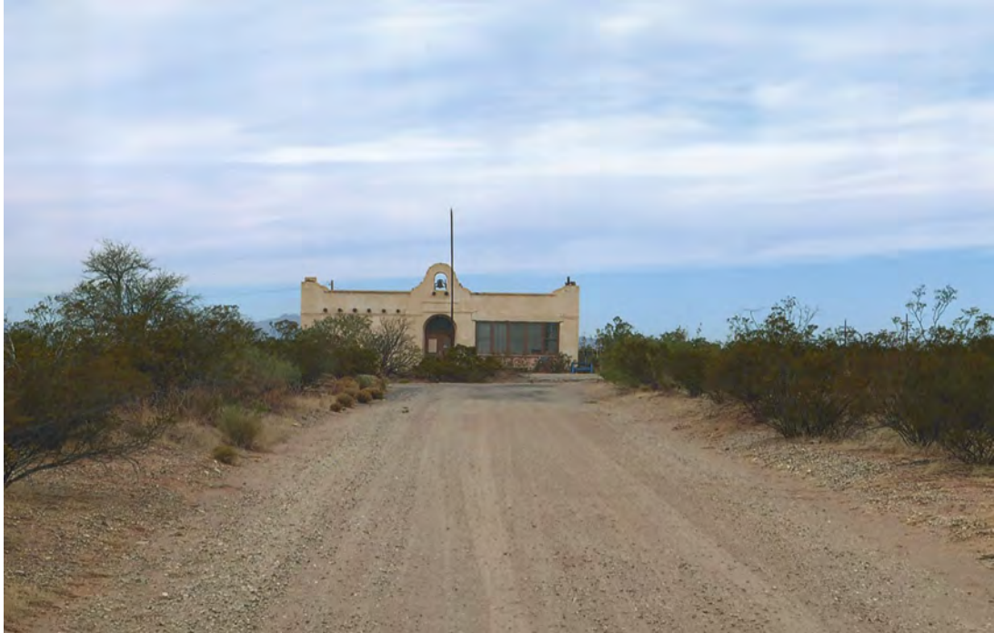
Orogrande School on Alabama Street, photographer facing west.
