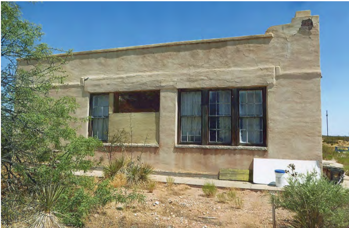
South side, photographer facing north.
