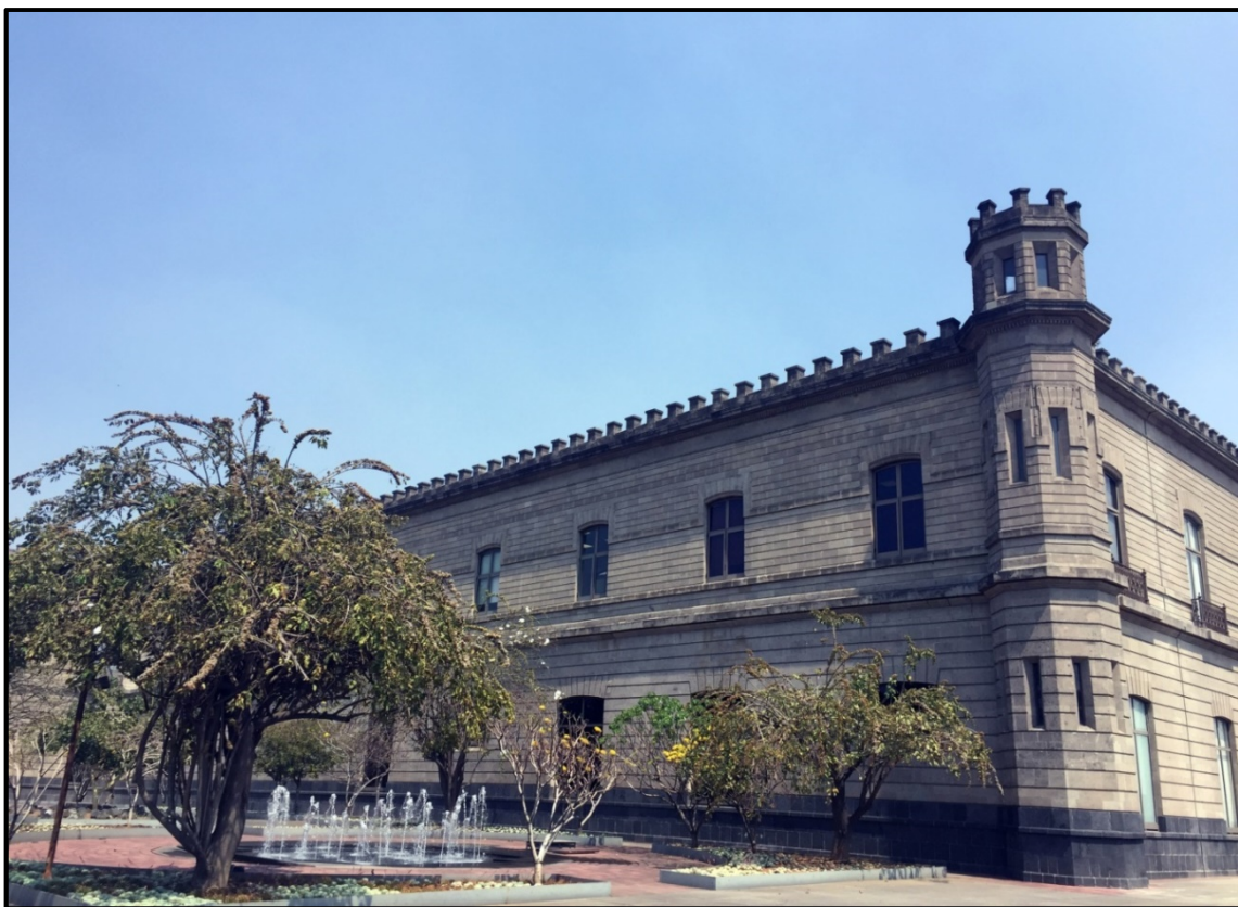
Photograph No. 1. The Palacio de Lecumberri, in Mexico City. The former prison now serves as a major repository for documents, maps, and many other items related to the history and governance of Mexico and other countries once part of New Spain, beginning with activities in Spanish Colonial times and continuing into the modern era. (Photograph by E.A. Oster).
