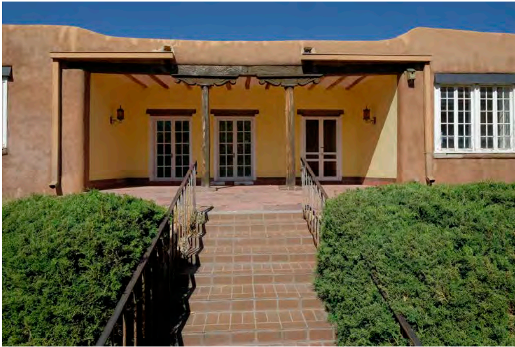
9 of 35. Detail, main entrance, photographer facing southwest.
