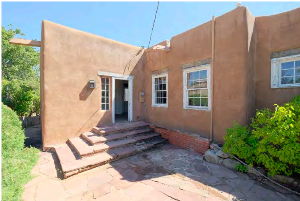
16 of 35. West side, kitchen entrance with carved lintels, photographer facing southeast.
