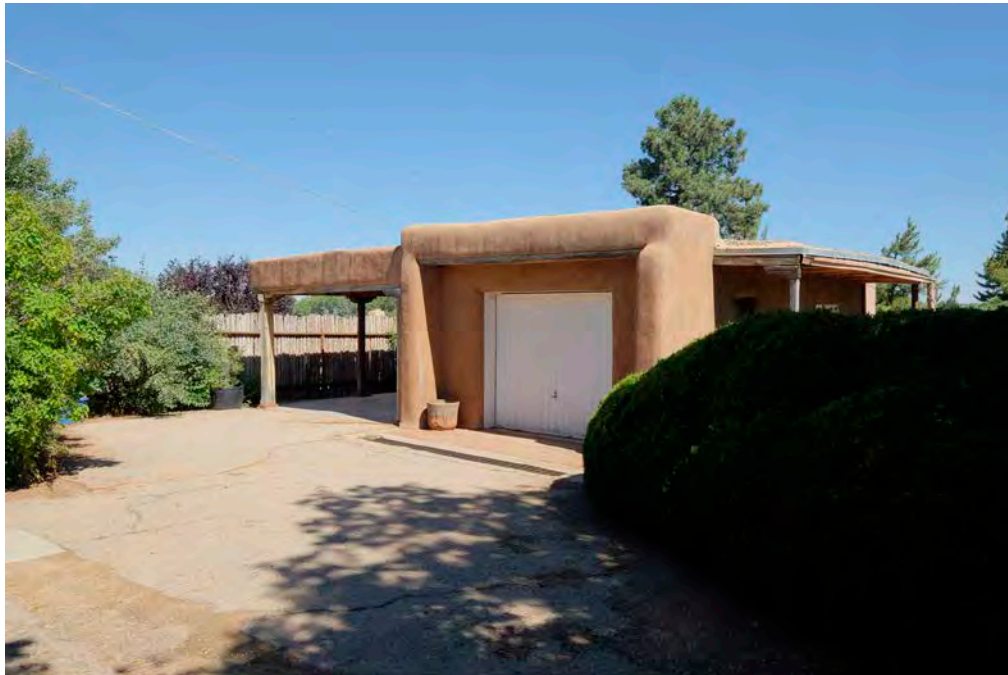
13 of 35. Garage, photographer facing southwest.
