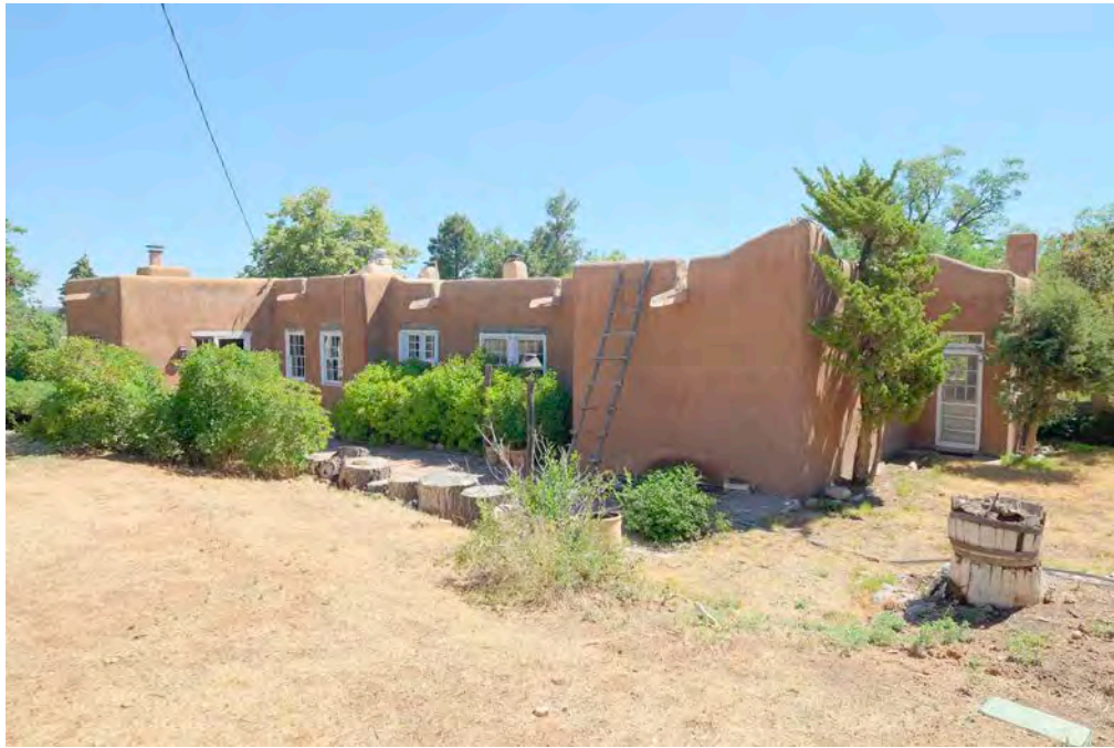
15 of 35. Rear (west) side of house, photographer facing southeast.
