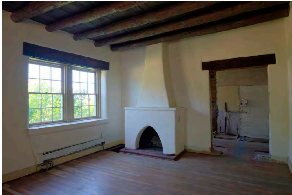
33 of 35. Interior, bedroom 1, photographer facing north.
