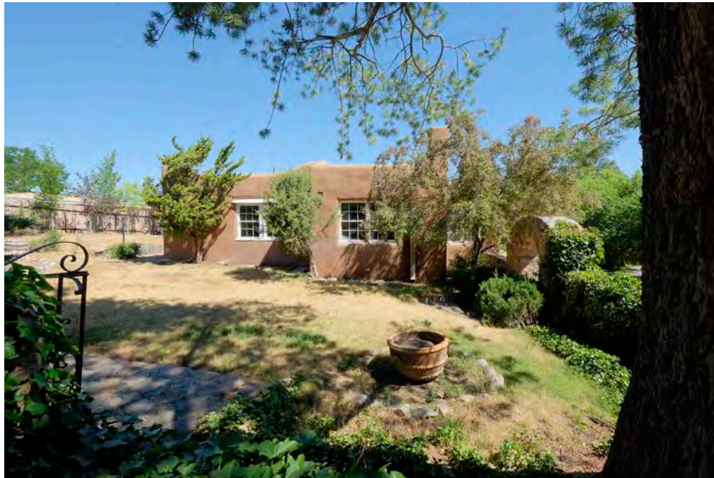
17 of 35. South side of house, photographer facing north.
