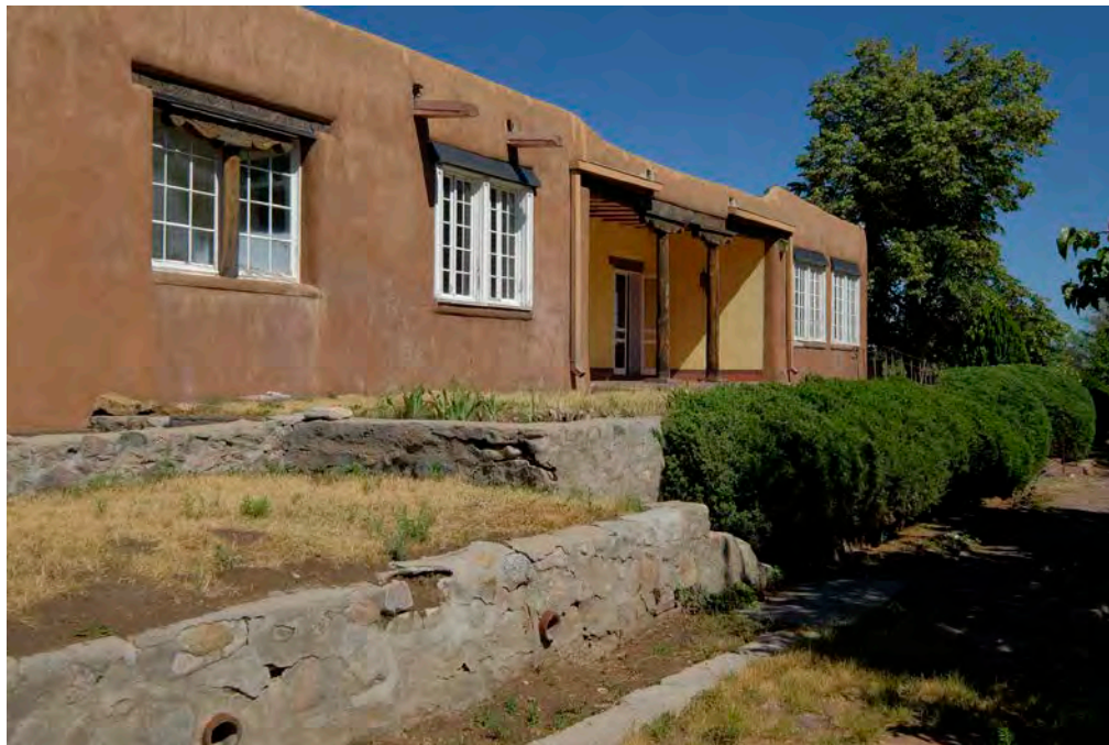
7 of 35. Main façade, photographer facing southwest.
