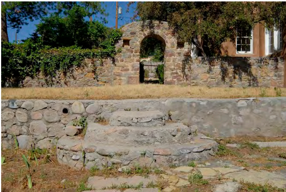
6 of 35. Stone stairs, retaining wall, and stone arch, photographer facing west.
