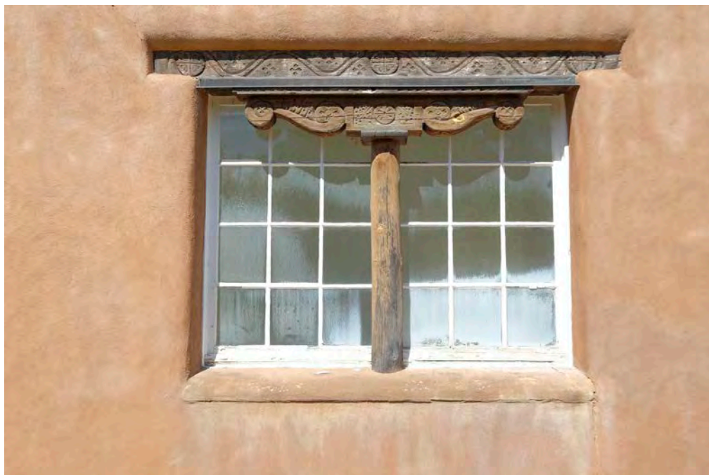
8 of 35. Detail, window with carved corbel and lintel, photographer facing west.
