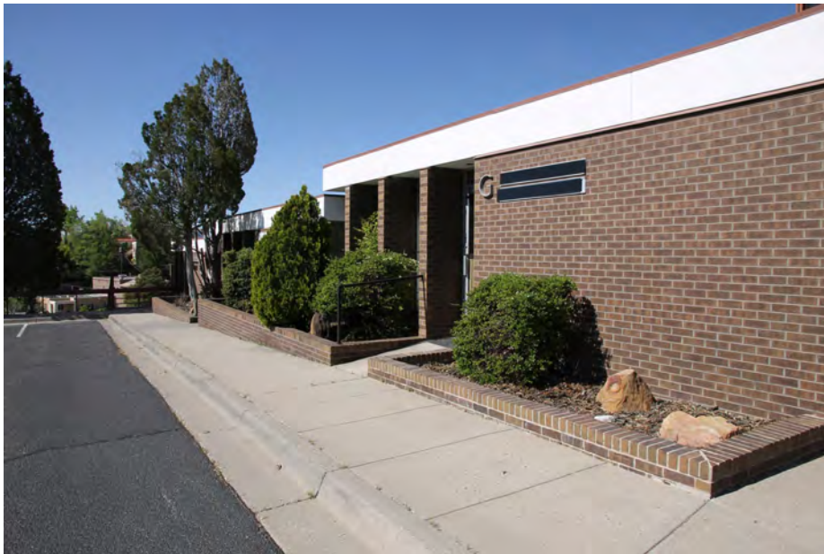
Granada Medical Plaza, west building, photographer facing southwest
