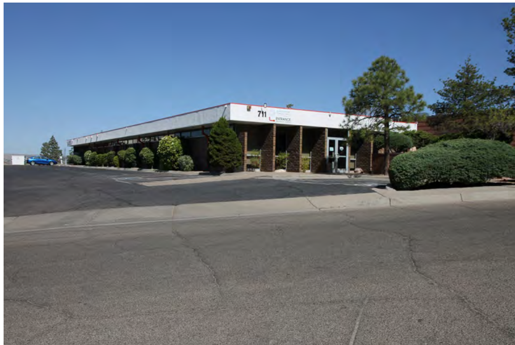
Granada Medical Plaza, north building, photogrpaher facing northeast
