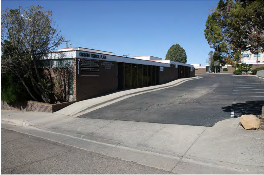
Granada Medical Plaza, south building, photographer facing southwest
