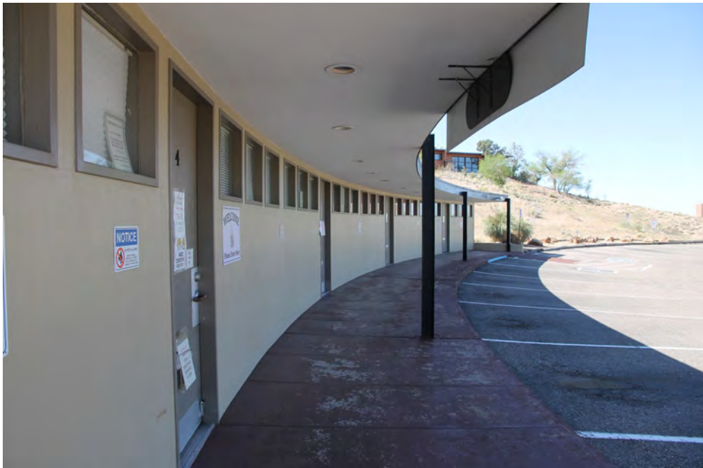
Encino Crescent, colonnade, photographer facing south
