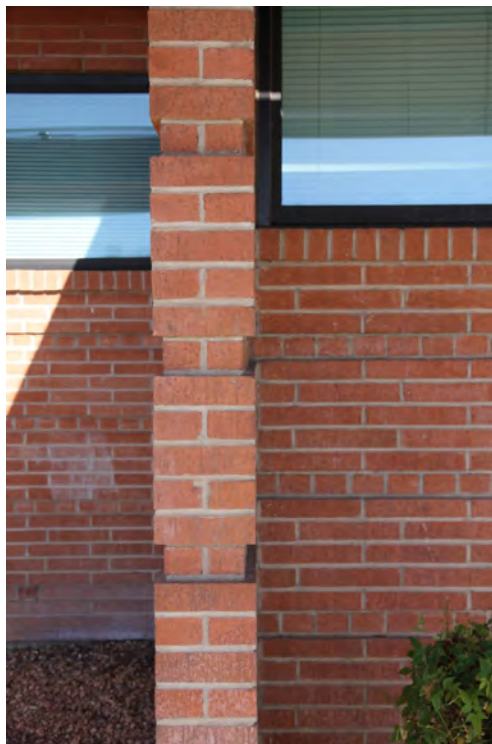
Encino Medical Plaza, masonry detail, photographer facing west
