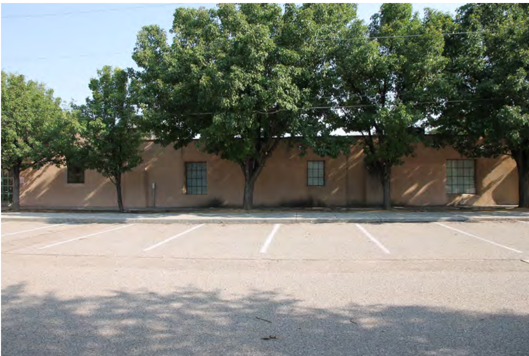
Photo 6. South façade, photographer facing north.
