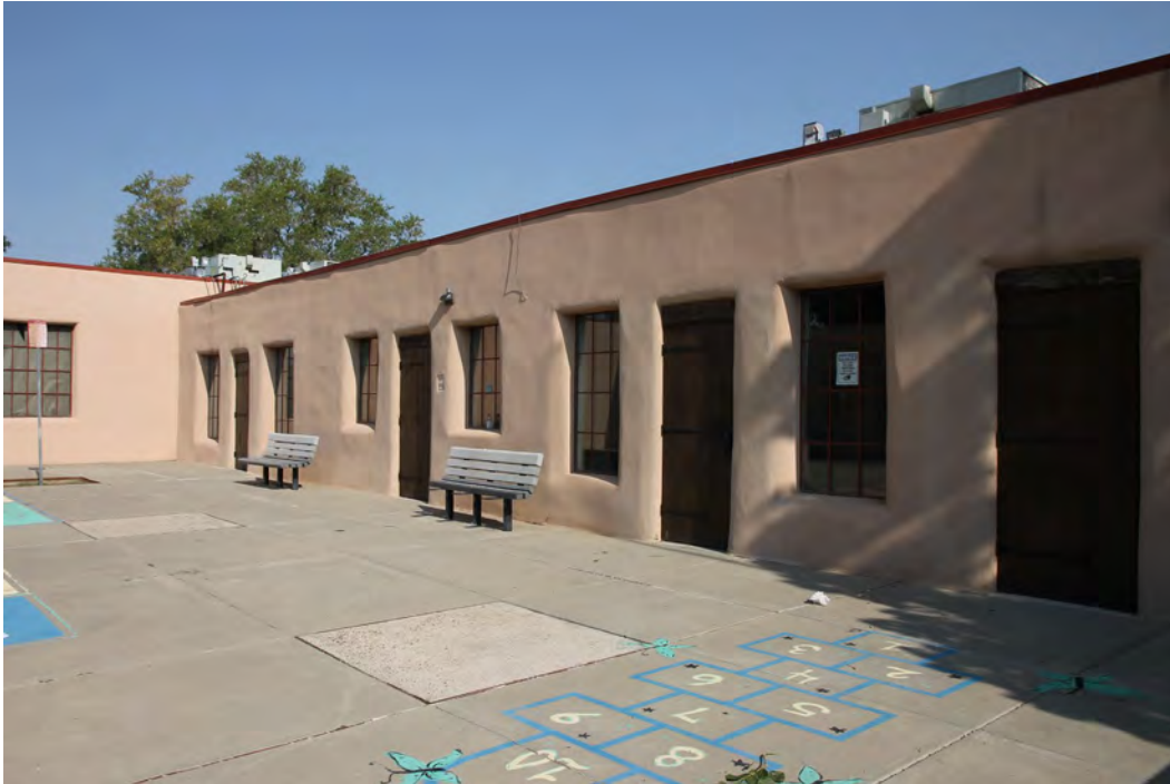
Photo 3. Courtyard, north façade, photographer facing northwest.
