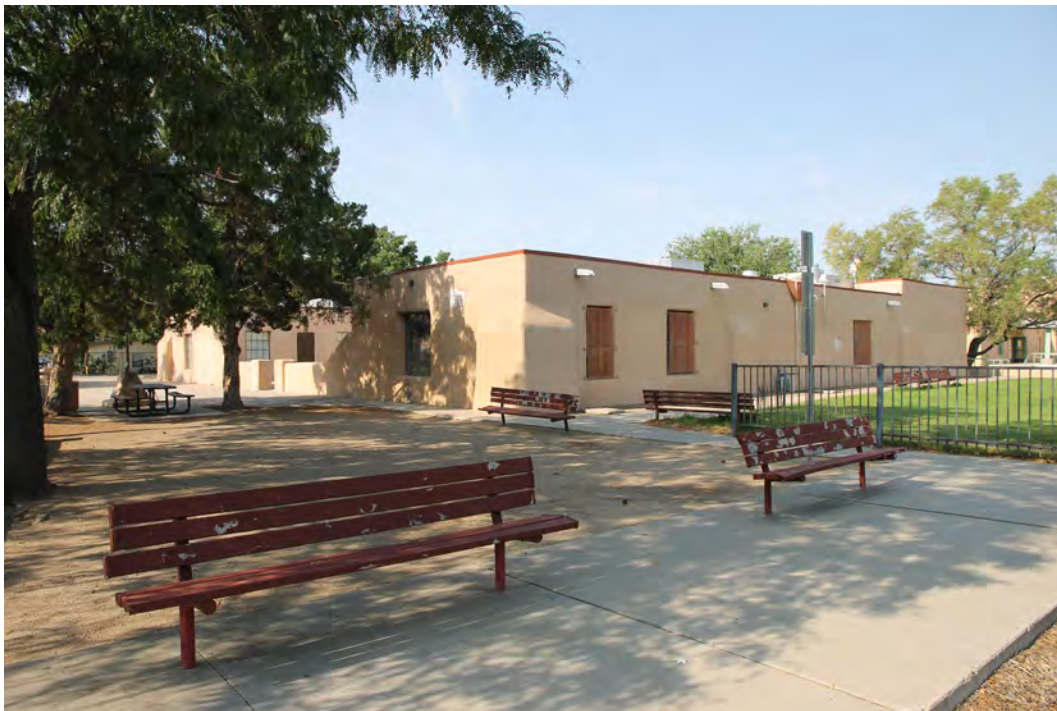
Photo 20. Plaza in front of Barelas Community Center, photographer facing southwest.
