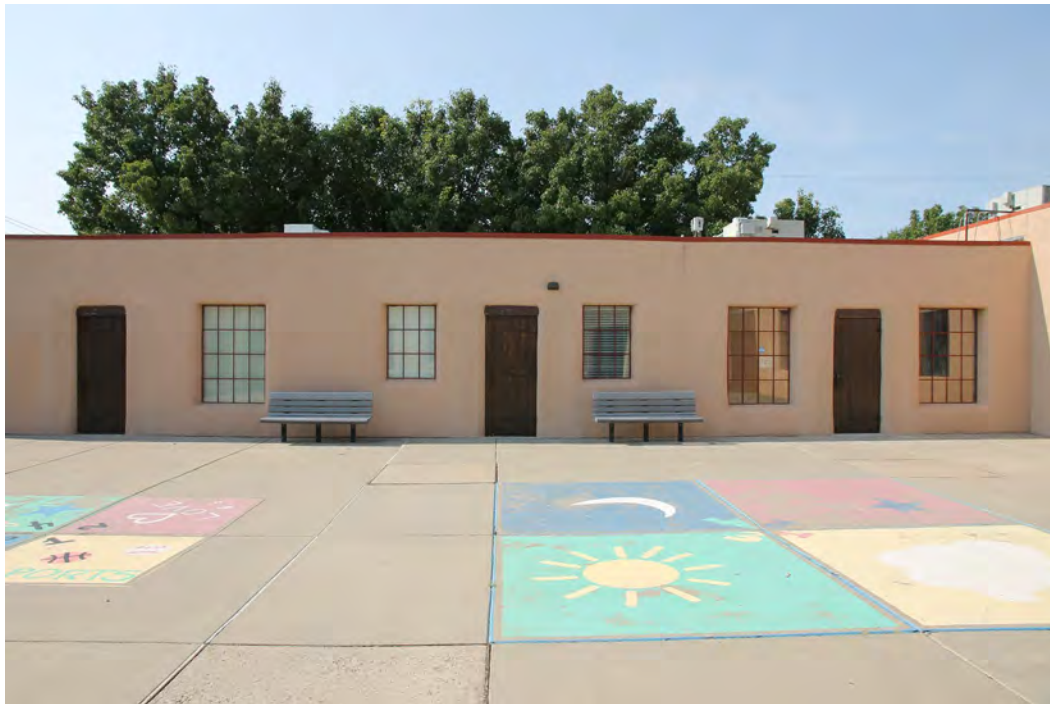
Photo 4. Courtyard, south façade, photographer facing south.
