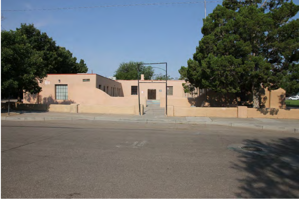
Photo 1. Main façade of Barelas Community Center, photographer facing west.
