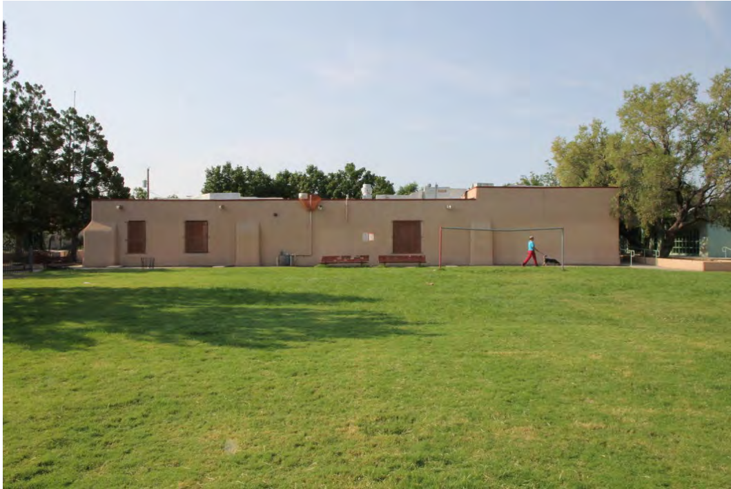
Photo 5. North façade, photographer facing south.
