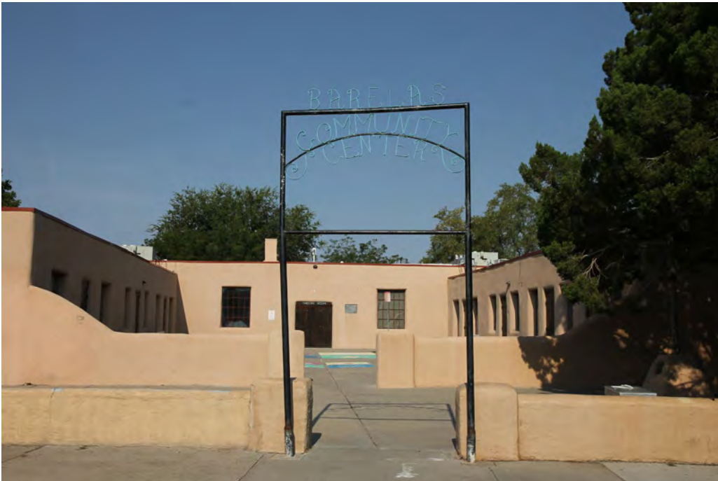
Photo 2. Entrance gate, adobe wall, courtyard, and main façade, photographer facing west.
