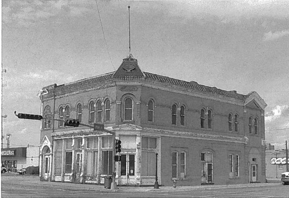
Photo 1 First National Bank/Carlsbad Irrigation District Building
