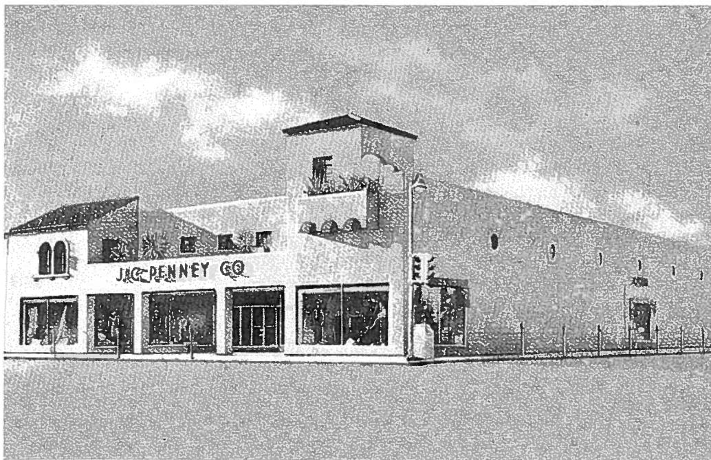
Figure 7.1 J.C. Penney Company Building
