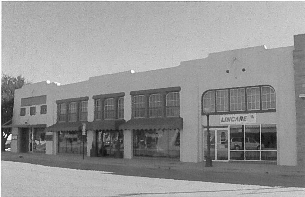
Photo 2 102-108 South Canyon St.
