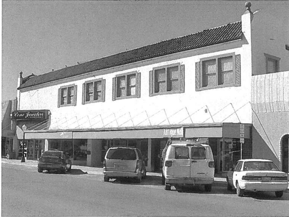
Photo 3 Former Cavern Theater, 105-111 South Canyon Street
