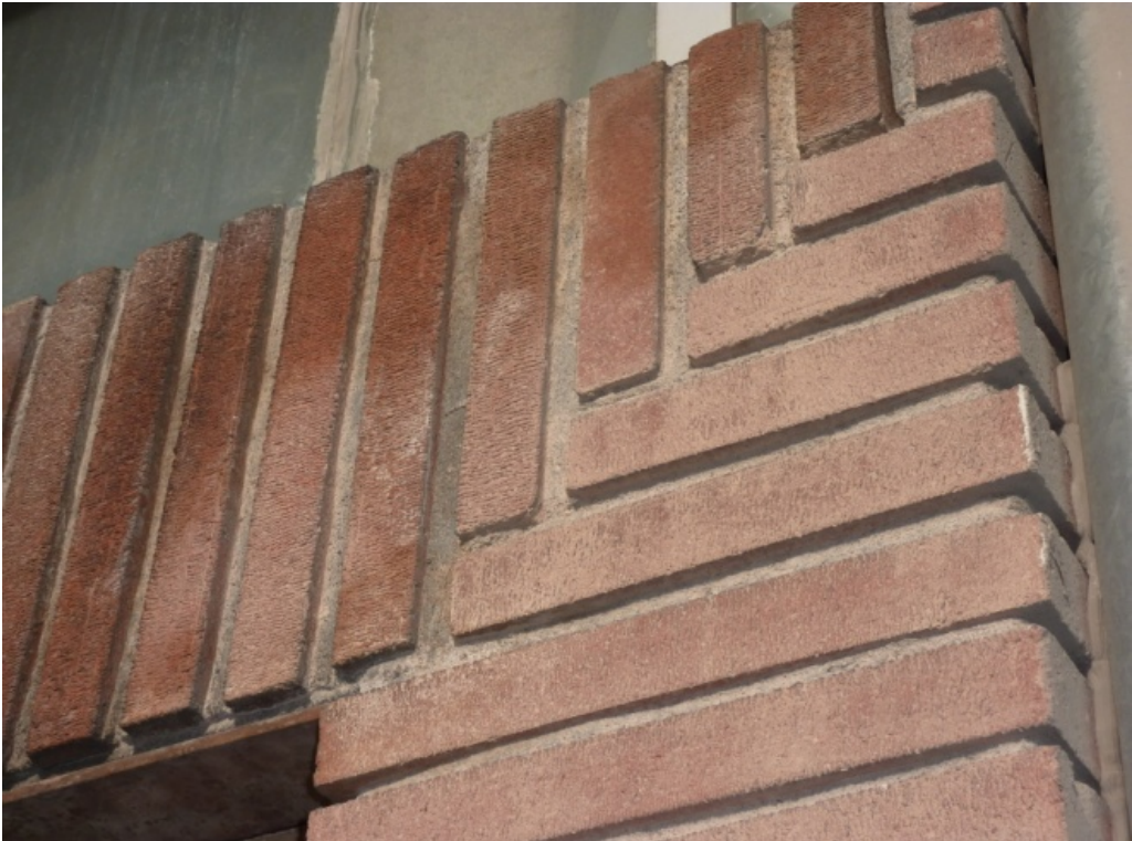
Photo 7: West elevation, brick border, front entrance, 2010
