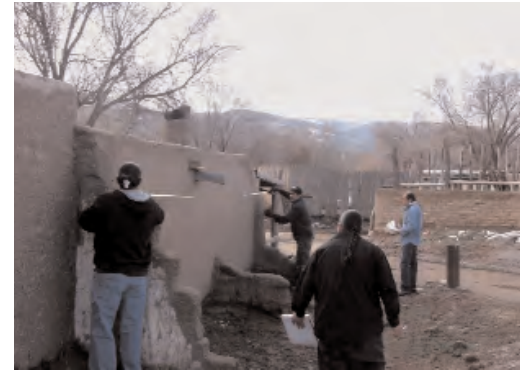
Pueblo residents formed a preservation crew and have begun the restoration.
