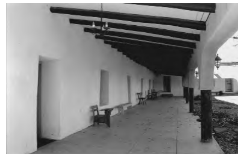
The veranda at Park Spring Ranch.
