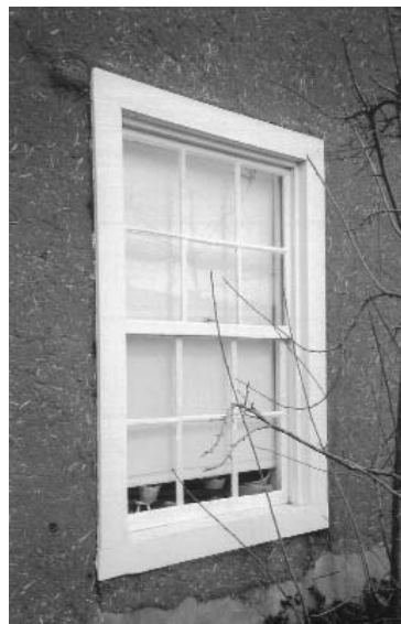
Windows were dismantled and rebuilt.
