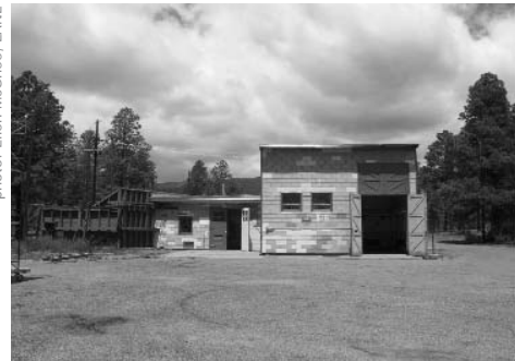
High Bay at V-Site.
