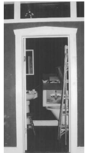
A rebuilt wall with original-style molding and a salvaged door inside.
