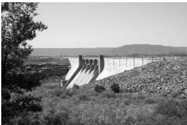
New Deal projects changed the face of New Mexico. Conchas Dam was the largest Depression-era construction project in the state.
