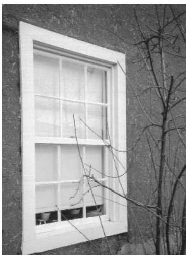
Windows were dismantled and rebuilt.
