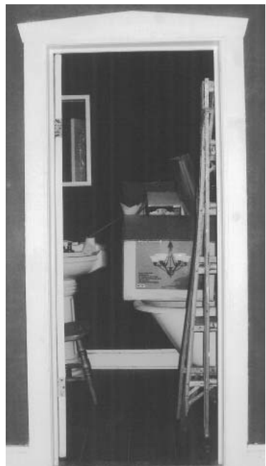
A rebuilt wall with original-style molding and a salvaged door inside.
