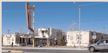
Demolition of the Aztec took two weeks in June.
