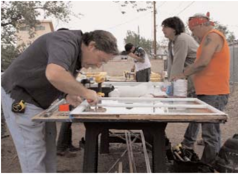
School founder Bob Yapp restores a window.
