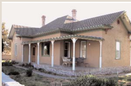
Constancio Mierra House in San Antonio was restored with state tax credits.
