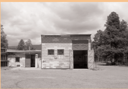
The restored High Bay Building. Notes, dates and formulas jotted down by scientists on its interior walls still can be read by visitors.
