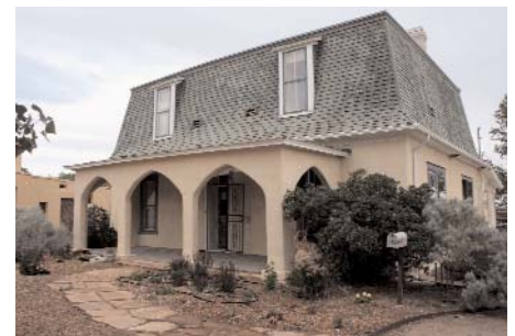
Built in 1903, the home was surrounded by orchards and market gardens at the edge of town. Constructed of adobe, it was a stand out with its shake-shingled, mansard roof.
